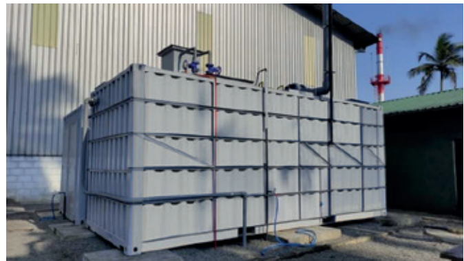
Puritas containerised sewage treatment plant
