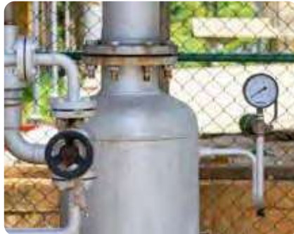
New flash vessel installation and condensate line resizing
