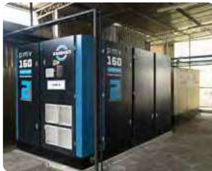
Reduce compressed air usage in the production department by commissioning of a new 160 KW Inverter type compressor to drive energy saving at the plant
