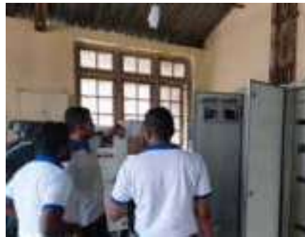
Energy Review conducted by NCPC
