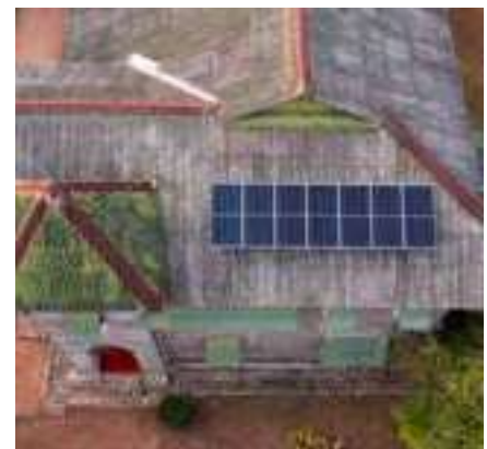
Off Grid Roof Mounted Solar
